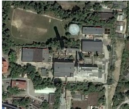
Exhibit 54: Chisinau CT-Sud Heat Boilers
