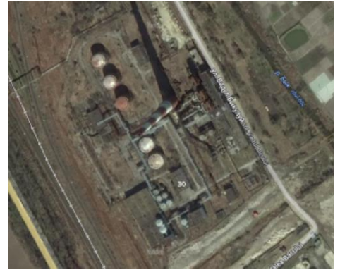
Exhibit 55: Chisinau CT-Est Heat Boilers
