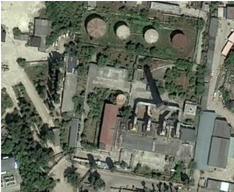
Exhibit 53: Chisinau CT-Vest Heat Boilers
